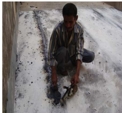
Photo 13: Thermosealing of the joints
