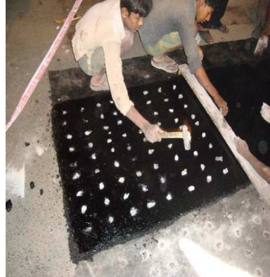
Photo 12: Placing of antiskid stone chips on masticated surface
