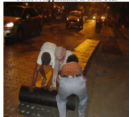
Photo 10: Laying of BJPF
