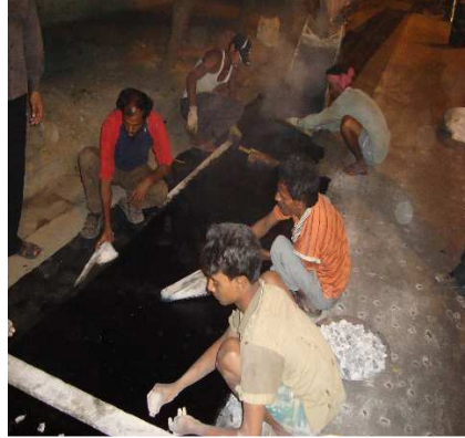
Photo 11: Laying of Mastic on BJPF
