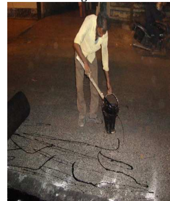
Photo 9: Application of Tack Coat
