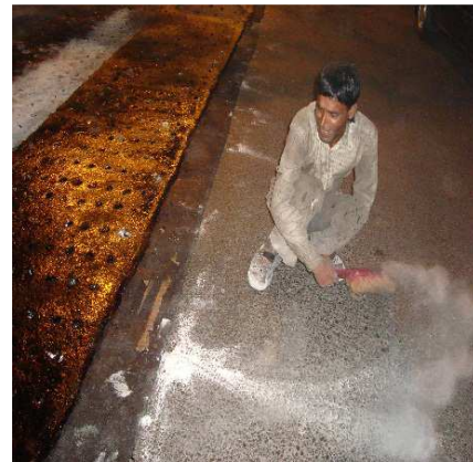
Photo 8: Cleaning of the road surface
